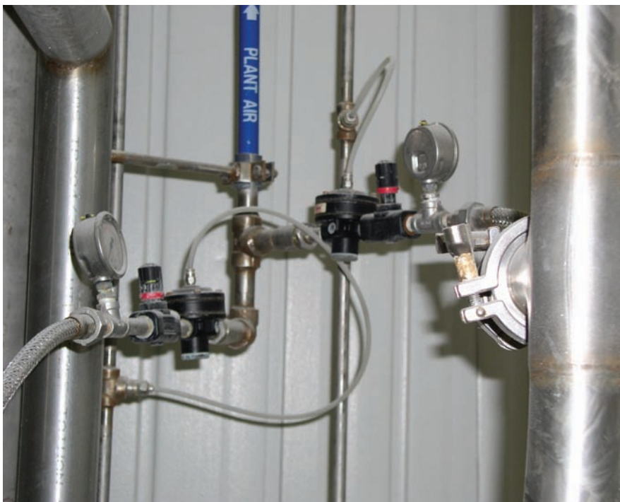
An air injector mounted in the conveying line helps move the salt through the line.
