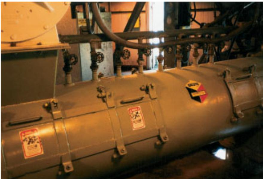
***The blender’s eight spray nozzles inject more than 200 gallons of recycled wastewater per minute and operate independently of each other.***
